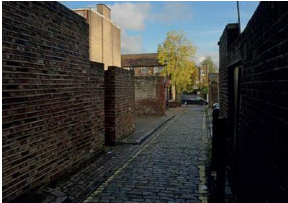
View of existing garages from Aquila Street (top) and view of garages looking east within Ordnance Mews (bottom).
