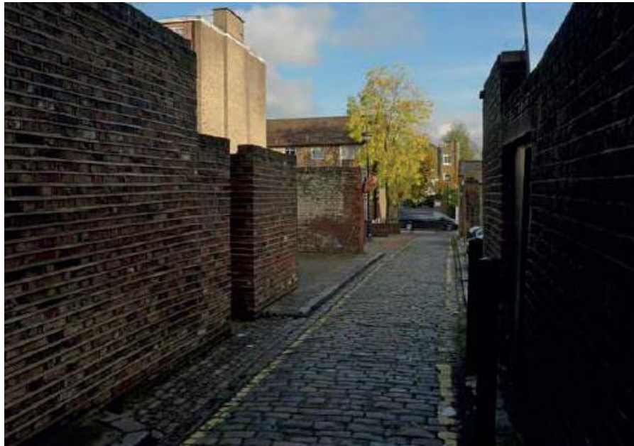
View of existing garages from Aquila Street (top) and view of garages looking east within Ordnance Mews (bottom).
